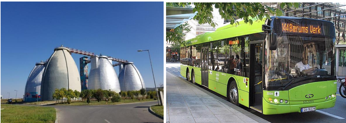
Figure 5: Anaerobic digestors in the APA NOVA WWTP (RO) and Oslo buses using biomethane.
